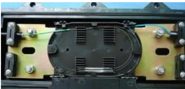
(4) Fix the weld fiber optics to the in-and-out port of the fiber splice and Put splice tray cover on.
